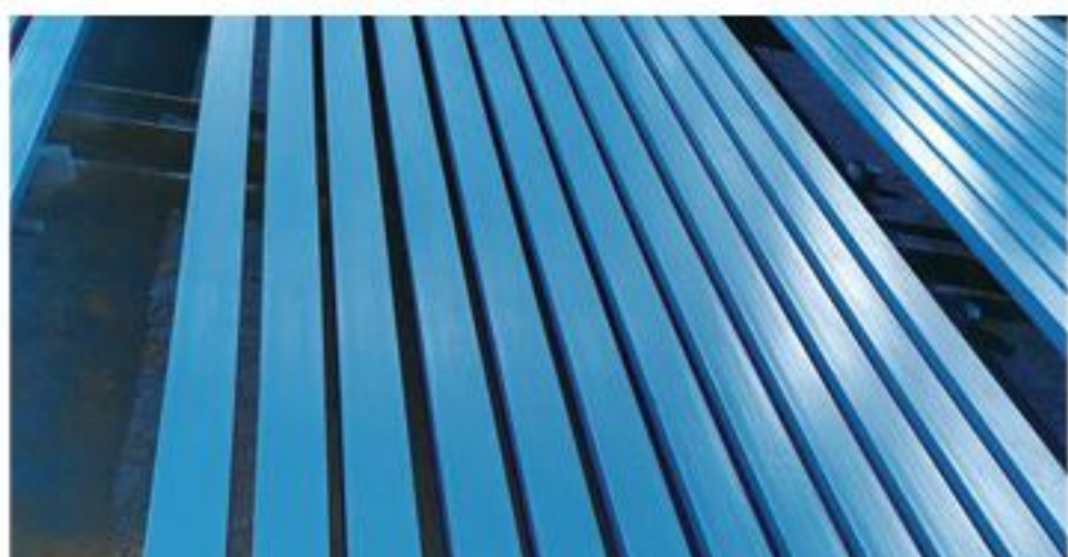
PAINTING Flat bar, steel plate, steel pipe, etc.
