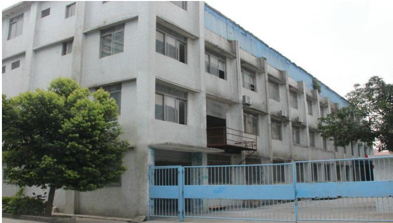
Factory Full View
