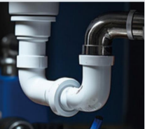
下水道疏通 Drain unclogging
