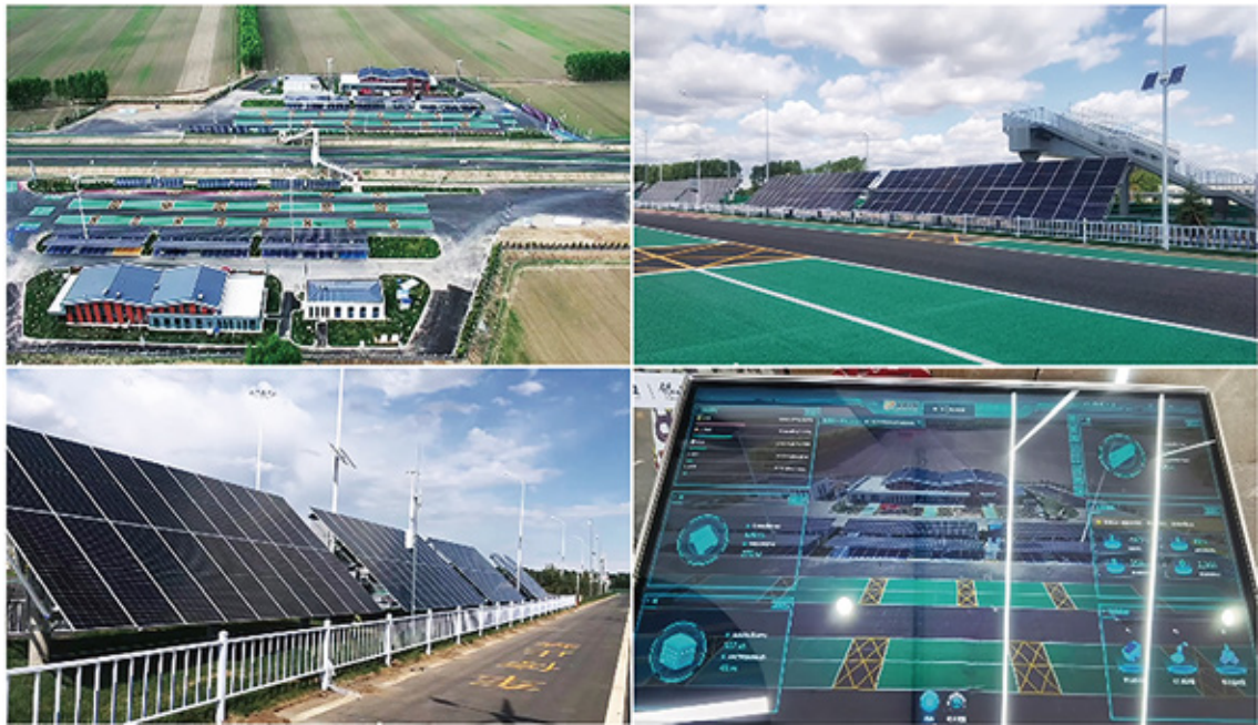
Heilongjiang Longjiang Transportation Province Expressway New Energy Project 7MW Project
