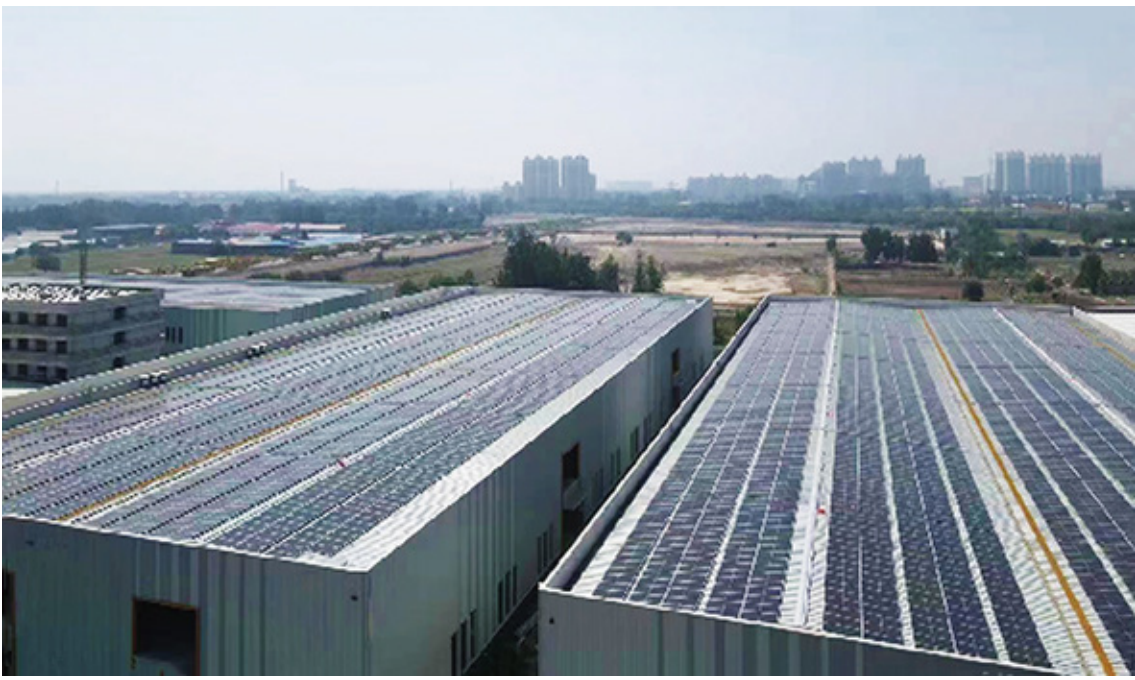
Shijiazhuang Huiao Cultural Communication Office Rooftop Distributed Photovoltaic Power Station 4.8MW Project
