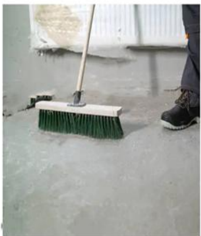
Step1 Cleaning Floor
