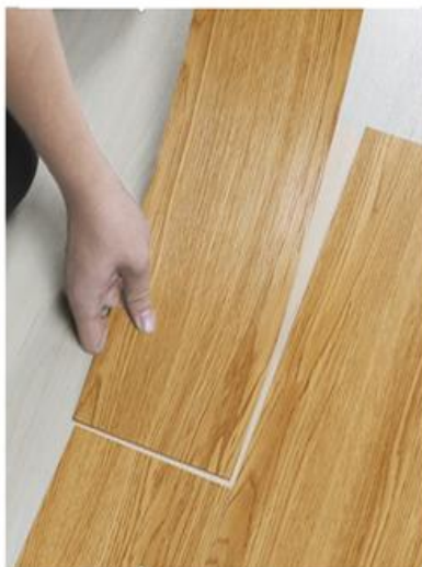
Step5 Install Flooring
