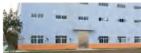
越南厂筹备中 VIETNAM PLANT IN PREPARATION
