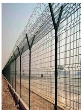
机场护栏 Airport fence
