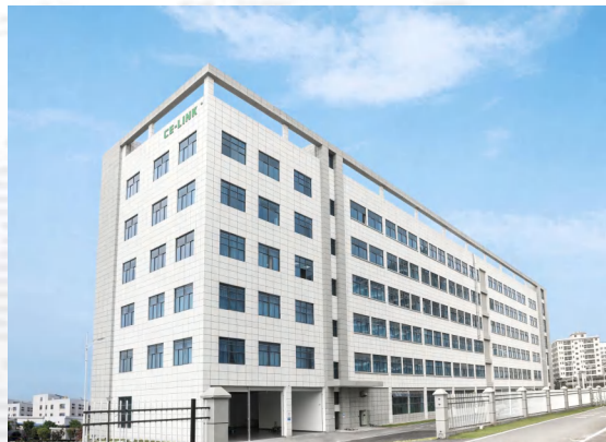
Battery cell production base
