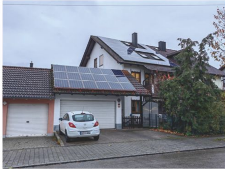
Stuttgart Germany 5kW+14.3kWh battery RESS
