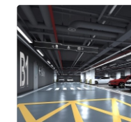
Parking lot lighting
