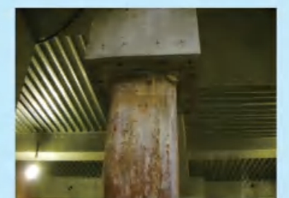
高层建筑基坑支护 High-rise building foundation
