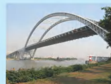
广州丫髻沙大桥 Guangzhou Yajisha Bridge
