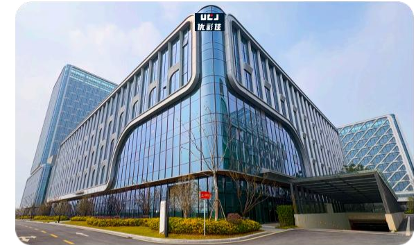
Anhui 16K m 2 NB, Soft Goods R&D and Assembly center
