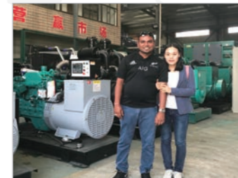
Cummins | 2017-11-04 Fiji Client @ Generator Factory
